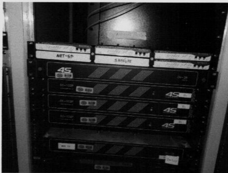
Vista do conversor SDI “Ensemble BrightEye 75” e codificador Pal-M “4S/EC-102P”
